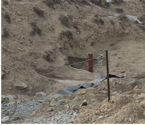
1#副坝下游扩散井
